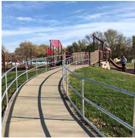
Ramp access to elevated play component structure
