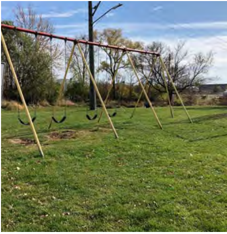
Swings at John's Park do not provide proper safety surfacing
