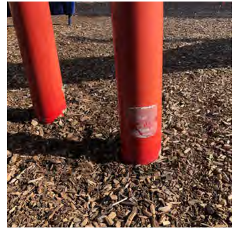
Remnants of safety surface level indicator sticker.
