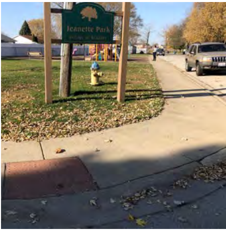
Existing crosswalk does not meet IDOT requirements
