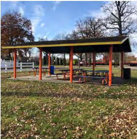
Picnic Shelter. Provide accessible route to shelter connecting to park entrances. Provide ADA picnic table.
