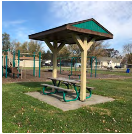
Covered picnic table. No accessible tables provided.
