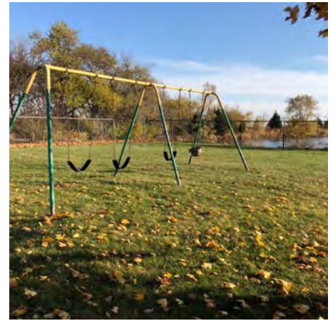
No safety surfacing at Swings
