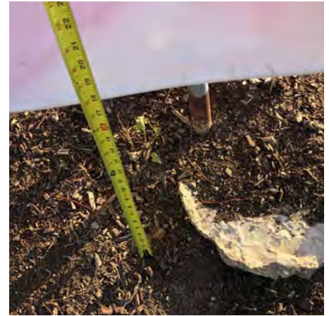
Safety Surfacing is too low for play equipment height requirements and impact attenuation requirements
