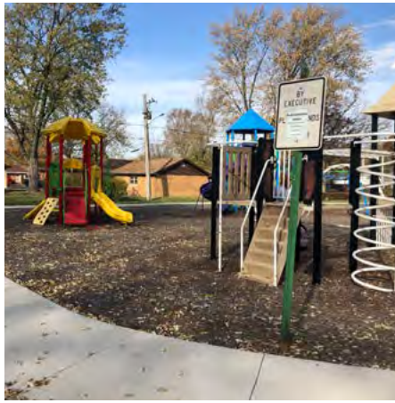
Playground includes 3 separate elevated component structures
