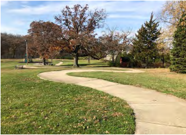
Park path follows a switch back pattern down the hill. Many sections of the path exceed 5% slope
