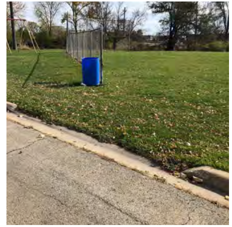
Park has no interior paths and there are no sidewalk connections
