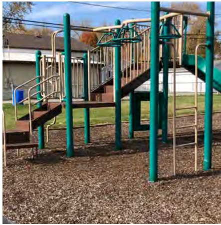
Elevated play component structure. Transfer station is provided.
