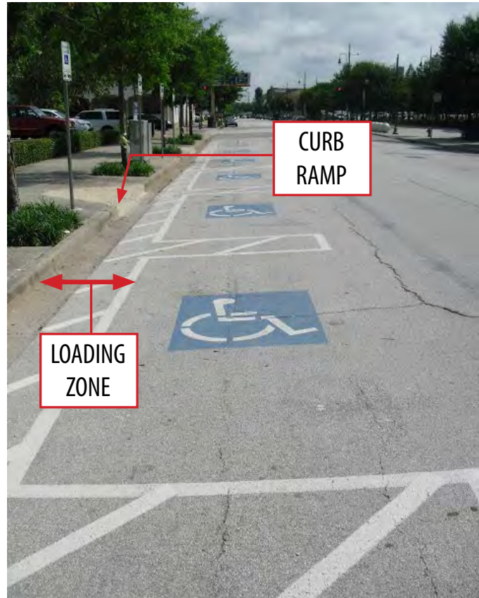
EXAMPLE OF ACCESSIBLE ON-STREET PARKING
