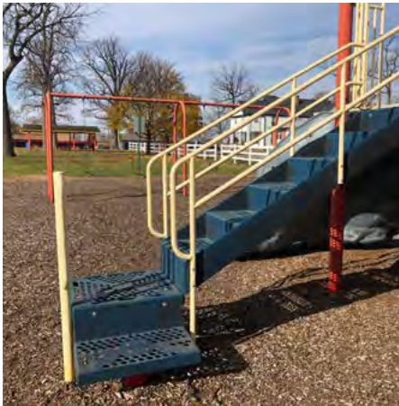
Transfer Platform at elevated play component structure
