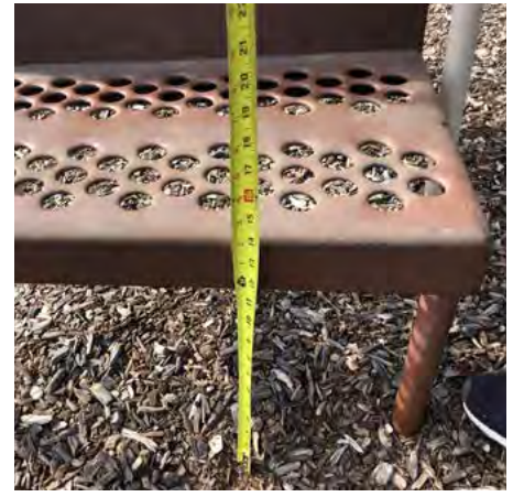
Safety surface level is too low relative to play equipment.
